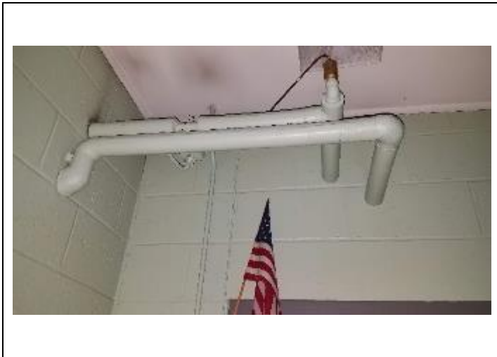
3. Typical ACM Pipe and Fitting Insulation located throughout building
