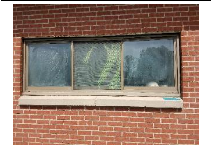
4. Sample locations 073018C05 (south side, center window, top header)
