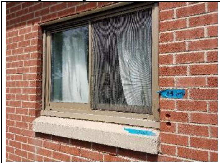
5. Typical windows with ACM trim caulk located throughout building
