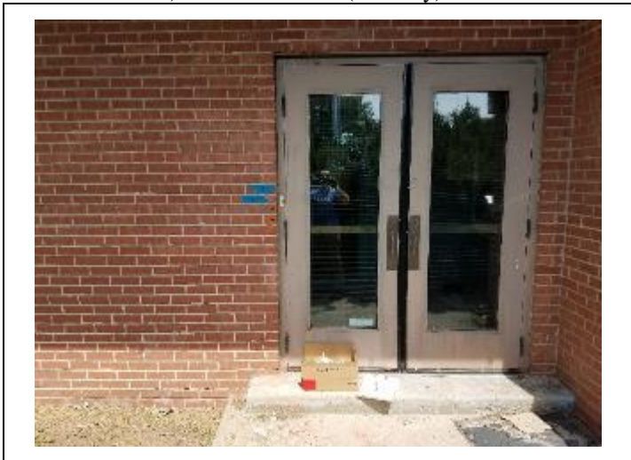
5. Sample location 073018C06 (south side, entry door, trim) and 073018C07 (masonry)
