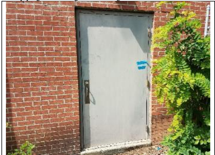
6. Typical door opening with ACM caulk at trim located throughout building
