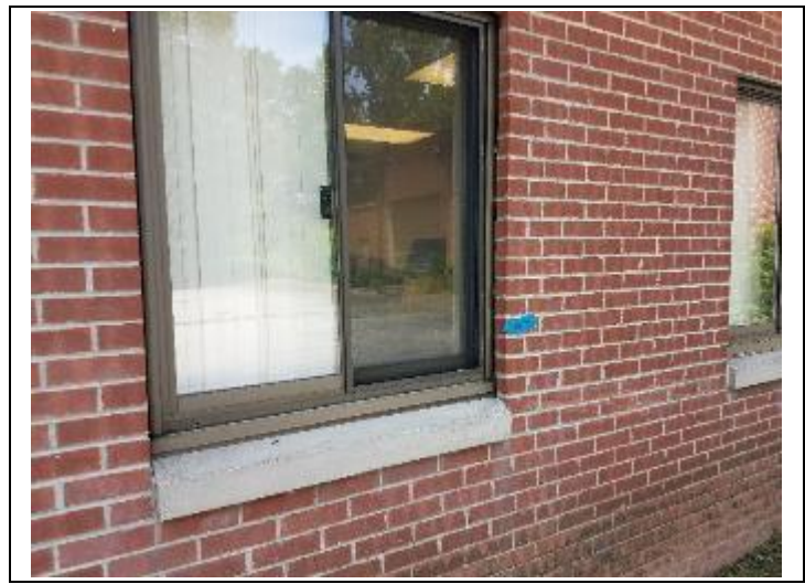
8. Sample location 073018C10 (north side, center office window, trim)
