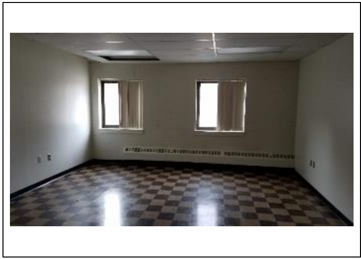
2. Typical ACM 9" Floor Tile and Black Mastic throughout
